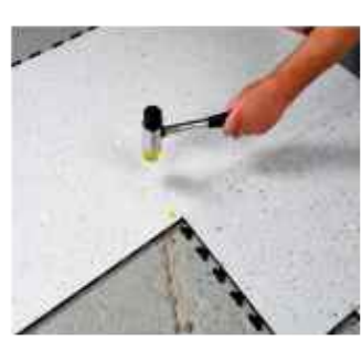
ESD Flooring Installation
